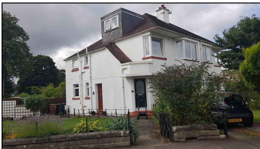
Fig 3 - View of apartment block from street. Entrance to No14 (upper floor flat) at front, and to No16 (ground floor) at side
